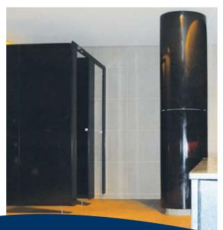
"The cladding panels were roll formed to fit the architects' design requirements as well as the actual site dimensions. As with all Vitraclad heavy gauge panels, the fabrication process takes place prior to enamelling. The raw materials of the product are smelted together in a kiln at approximately\_1200°C for four hours and then rapidly cooled," says Cottino.
